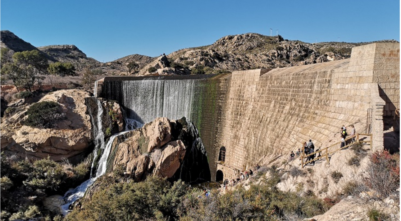
Elche Dam (XVII century)
