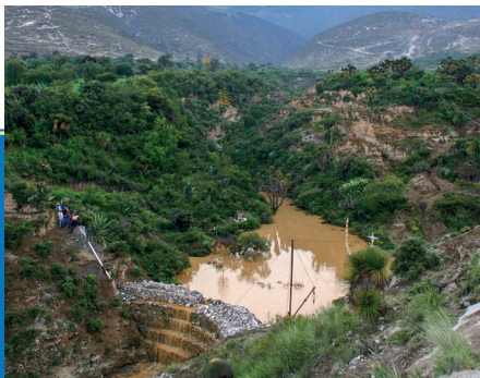
Traditional rock dams filter water and simultaneously allow infiltration. © Raúl Hernández Garcíadiego.
